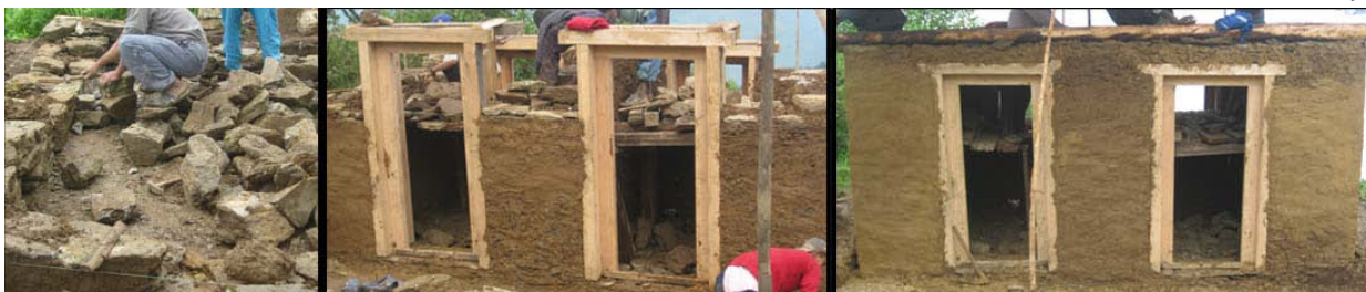
Construction of Toilet and Shower
